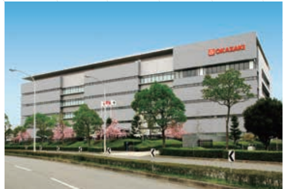
Main Manufacturing Factory
