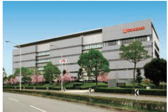
Main Manufacturing Factory
